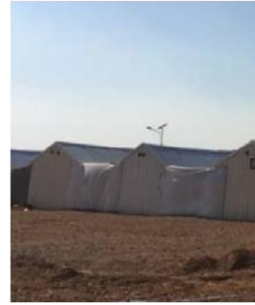
Fig. 22 Enclosed outdoor area [15]
