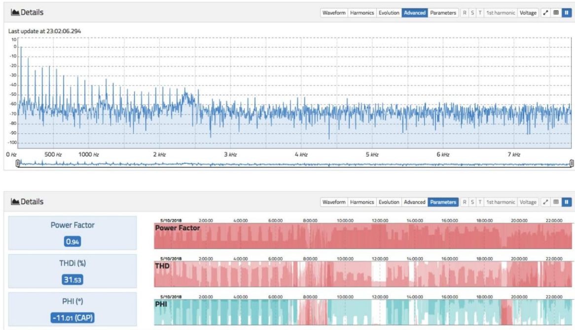
Figure 12. Top: current spectrum. Bottom: advanced parameters THDi, power factor, and phase angle for current.
